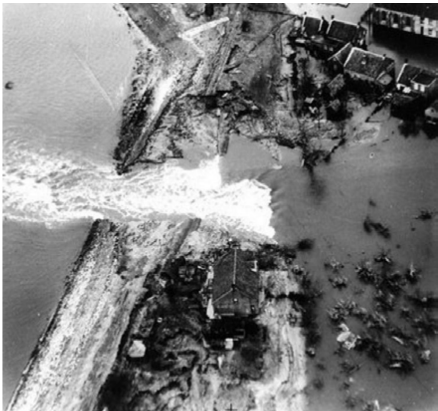
Dike breach during the North Sea flood of 1953
